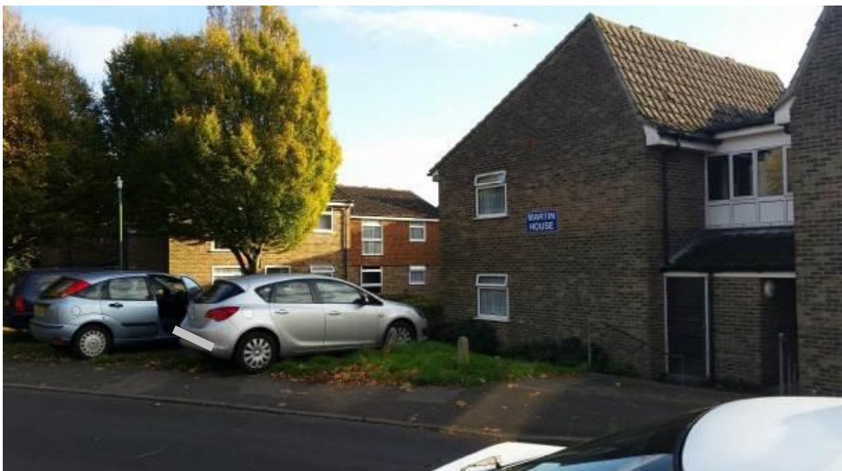
Figure 9 - Expanded view of northern elevation facing onto Little Chequers.
